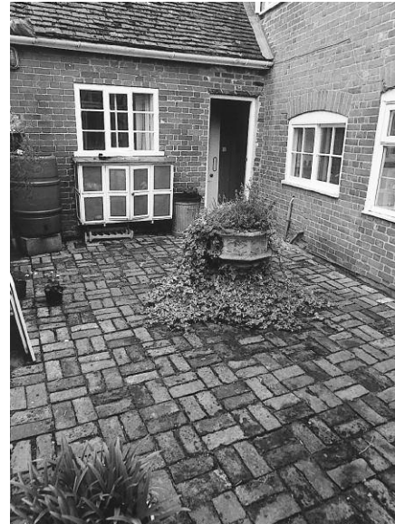
The new patio at Kersey Mill, with the original Suffolk bricks from the Yard re-used
