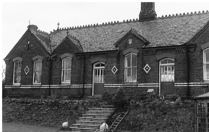
Old Isolation Hospital, now a dwelling
